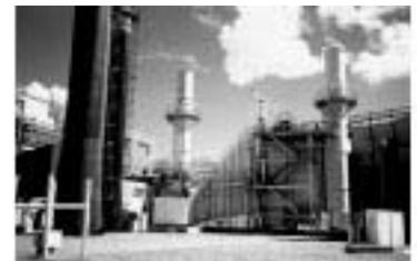
The Combined Cycle Turbine(25,800 kW) at the Animas Power Plant was completed in 1994 and fully operational, using state-of-the technology design, netting 38% more efficiency than the plant's next best generator.
